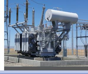
Transformers are key and expensive components of the electrical grid and knowledge of their health condition is essential to having a reliable network. When a transformer's insulation system is overstressed, gases are produced that dissolve in the oil. Dissolved Gas-in-oil Analysis (DGA) is recognized as the best indicator of developing faults in a transformer.
