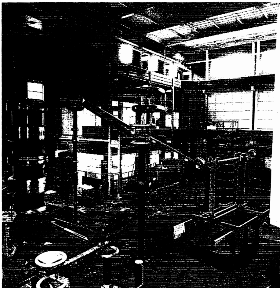
Figure 1b the disconnector during the RIV test on June 20, 1990, in the High-Voltage Laboratory of N.V. KEMA, Arnhem, the Netherlands. (KEMA photograph no. 902-0266/15.)
